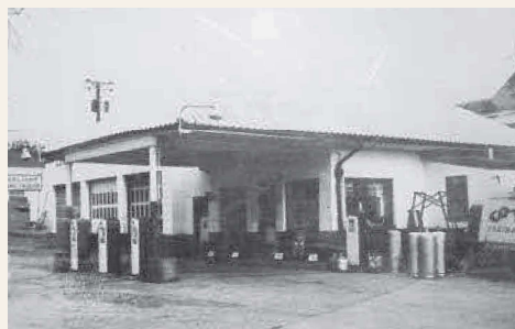
This photograph of the Community Co-op store is from the late 1950s. The cooperative convenience store is at the same location on Division Street today.
